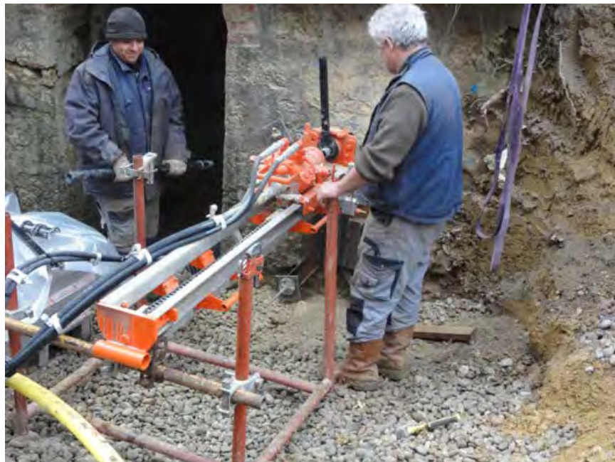
Figure 2.1.4.2 - Steunick BBAS pneumatic drill mast
