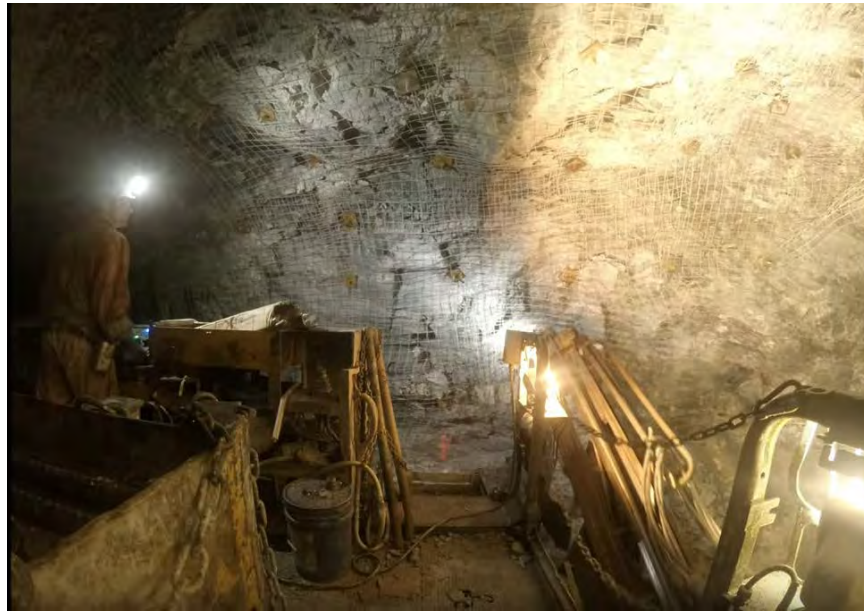
Figure 2.1.4.3 - Maclean scissor bolter operation
