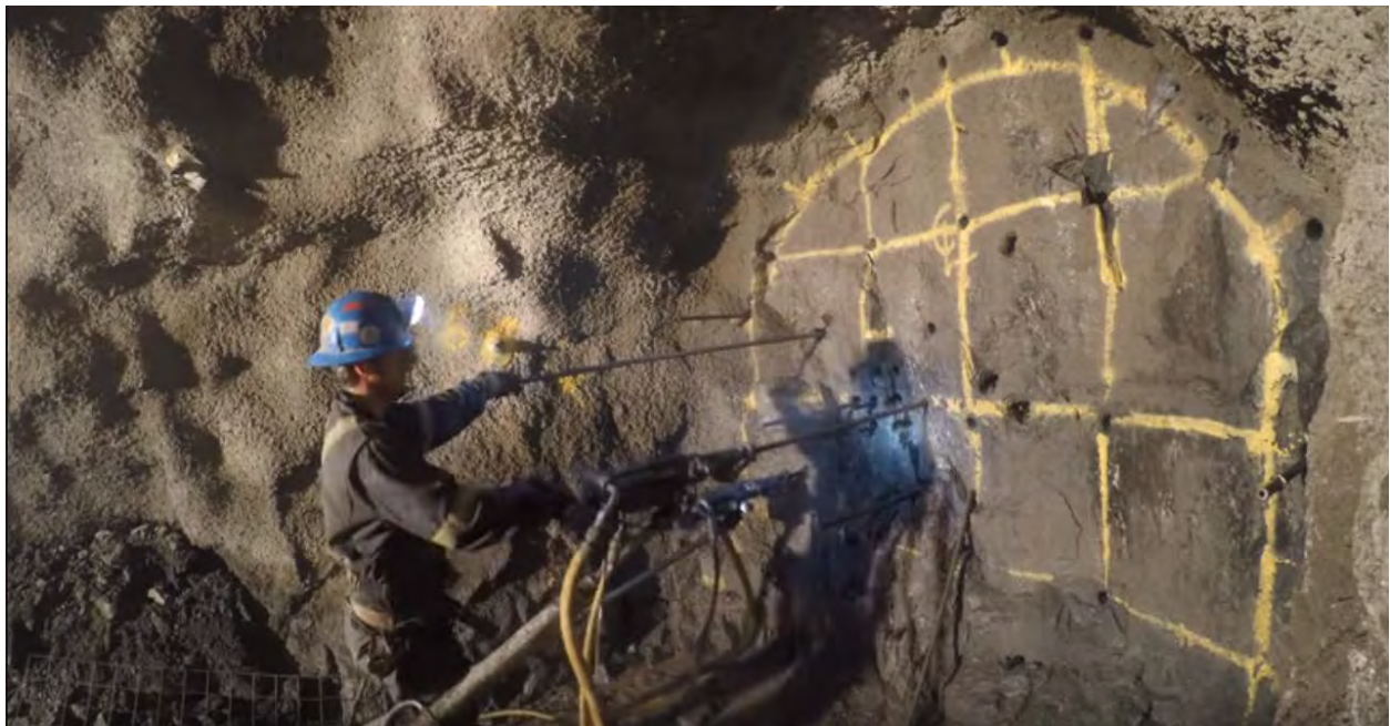
Figure 2.1.4.6 - MWS83 drill operation
