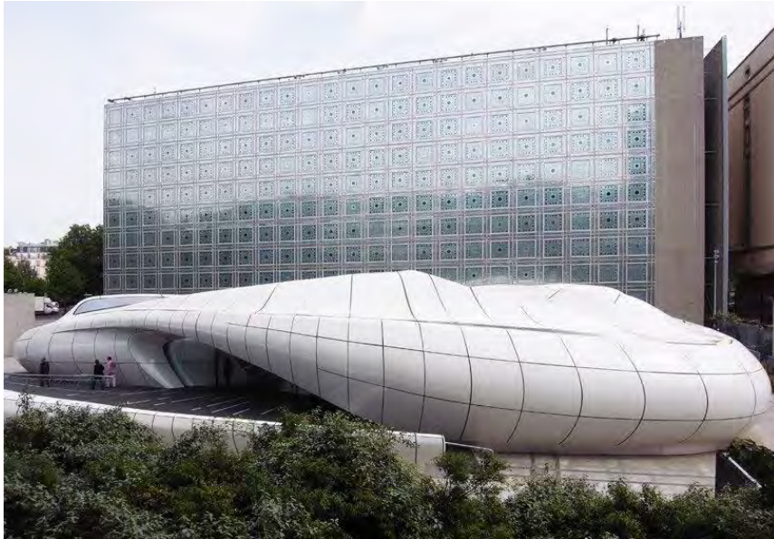
Figure 8 - Chanel Mobile Art Pavilion made of FRP or GRP (glass Reinforced plastic) exterior and interior structure by Architect Zaha Hadid.
