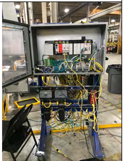
Example #3 of a PLC control (mobile)
