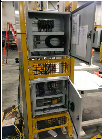
Example #2 of a PLC control
