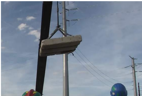
3. Removing large slabs with rigging
