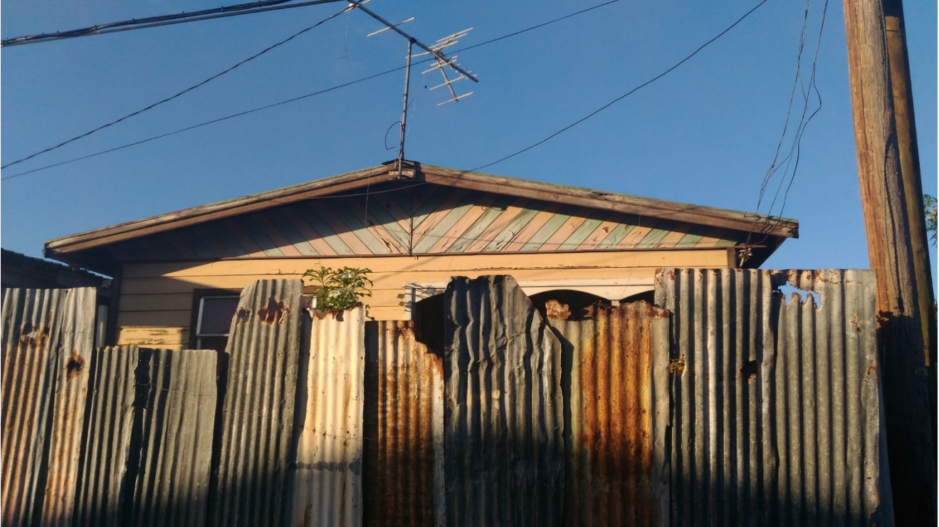
Figure 14. Traditional Barbadian vernacular architecture showing the use of 'galvanise' as a fence or wall
