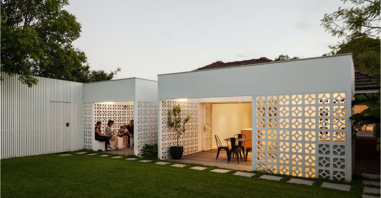
Figure 15. Breezeblocks used to create outdoor space
