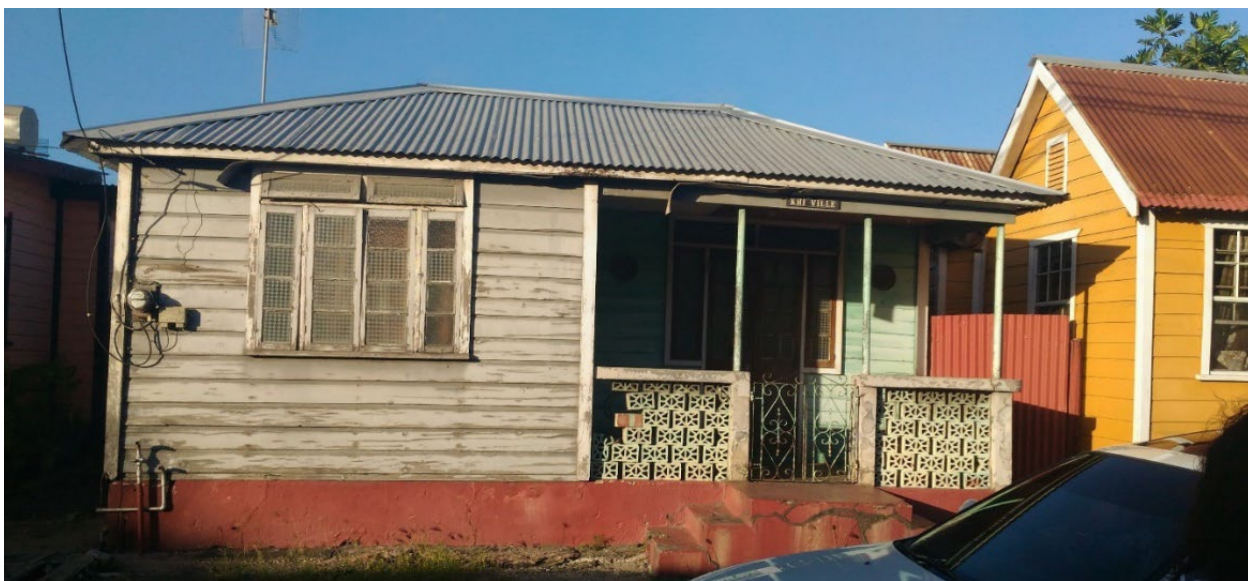
Figure 13. Traditional Barbadian Vernacular Architecture
